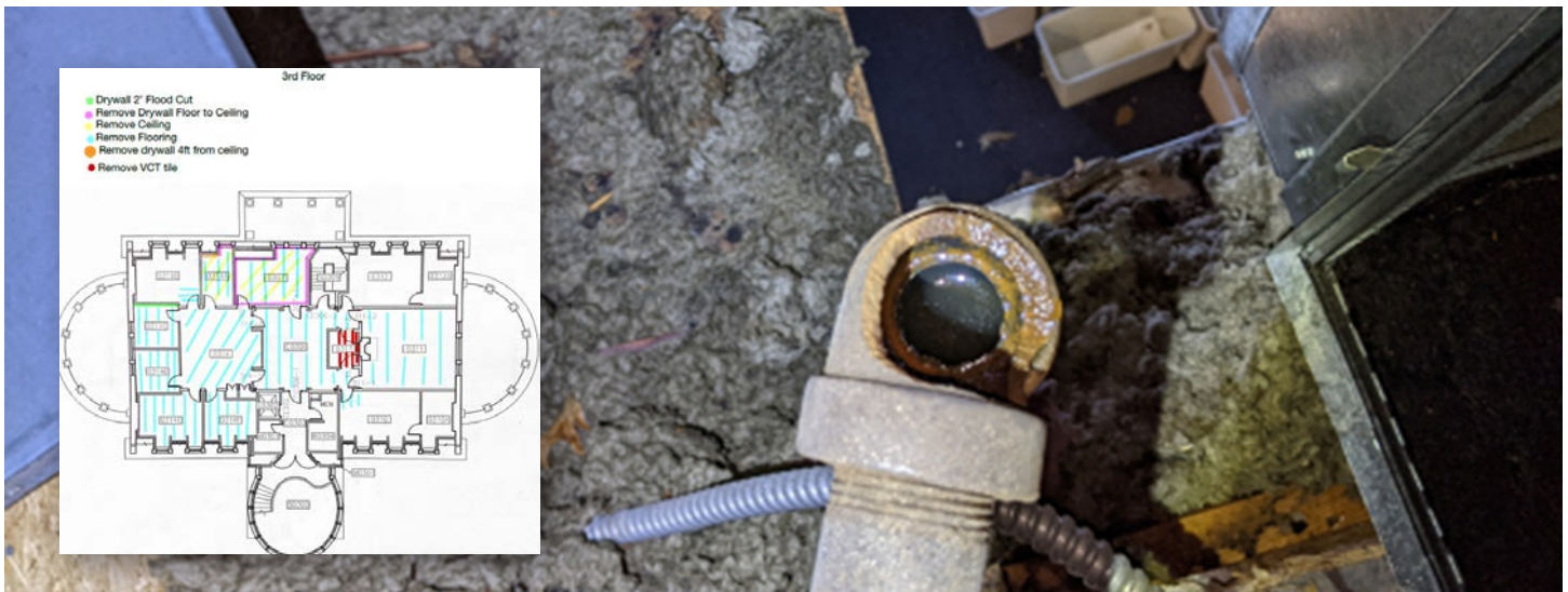
Map of demolition plans for the third floor of the Enrollment Services Center overlays a photo of the broken sprinkler fitting above room 307. Photo taken looking down from the attic.
