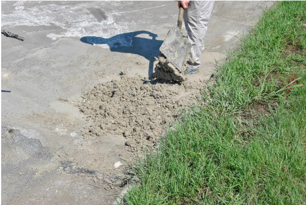
Solidification of concrete slurry
