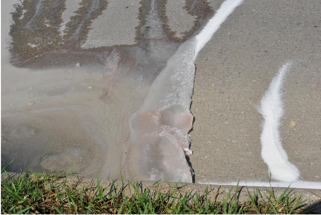
The super absorbent begins the solidification process
