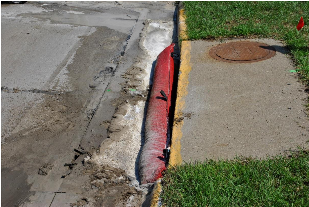
The super absorbent protects a storm water intake
