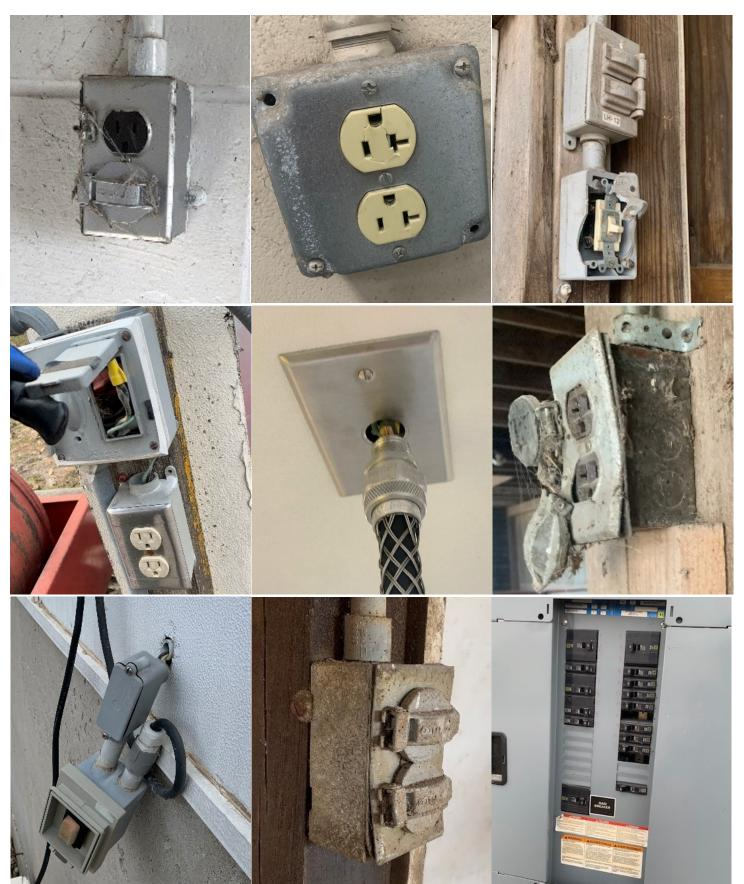
outlet cover plate. Open spaces in panel missing blank covers.
