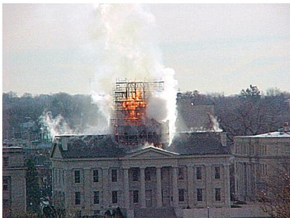
A fire in 2001 destroyed the dome of Iowa's historical Capitol building in Iowa City because of a failure to follow proper hot work procedures.
